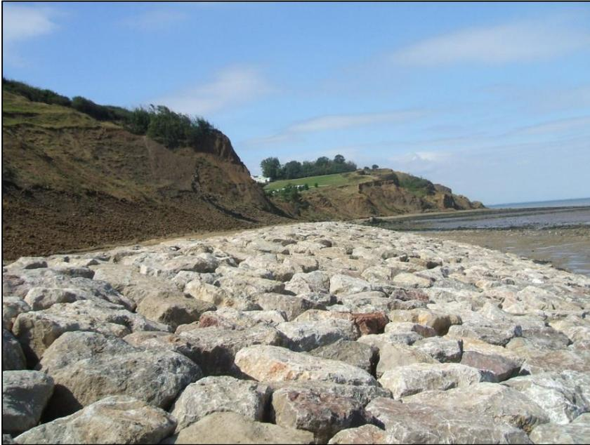
**Revetments** - Onshore sloped structures used to reduce the landward migration of the beach due to coastal erosion. Wave energy is limited by the structure to reduce the erosive power of the wave action. They can be constructed out of concrete, stone or asphalt. The structure should be designed to have a crest sufficiently high to stop wave overtopping during a storm event. The diagram below shows a recently constructed rock revetment at Warden Bay.
